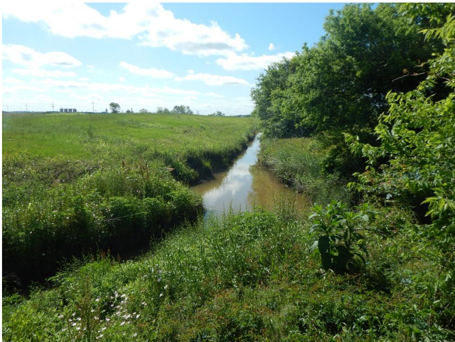
Photograph 4. The photo was taken at lat/long: 30.06342, -94.32152 facing southeast down the channel. The JCDD6 is proposing to widen the channel to improve conveyance and drainage.
