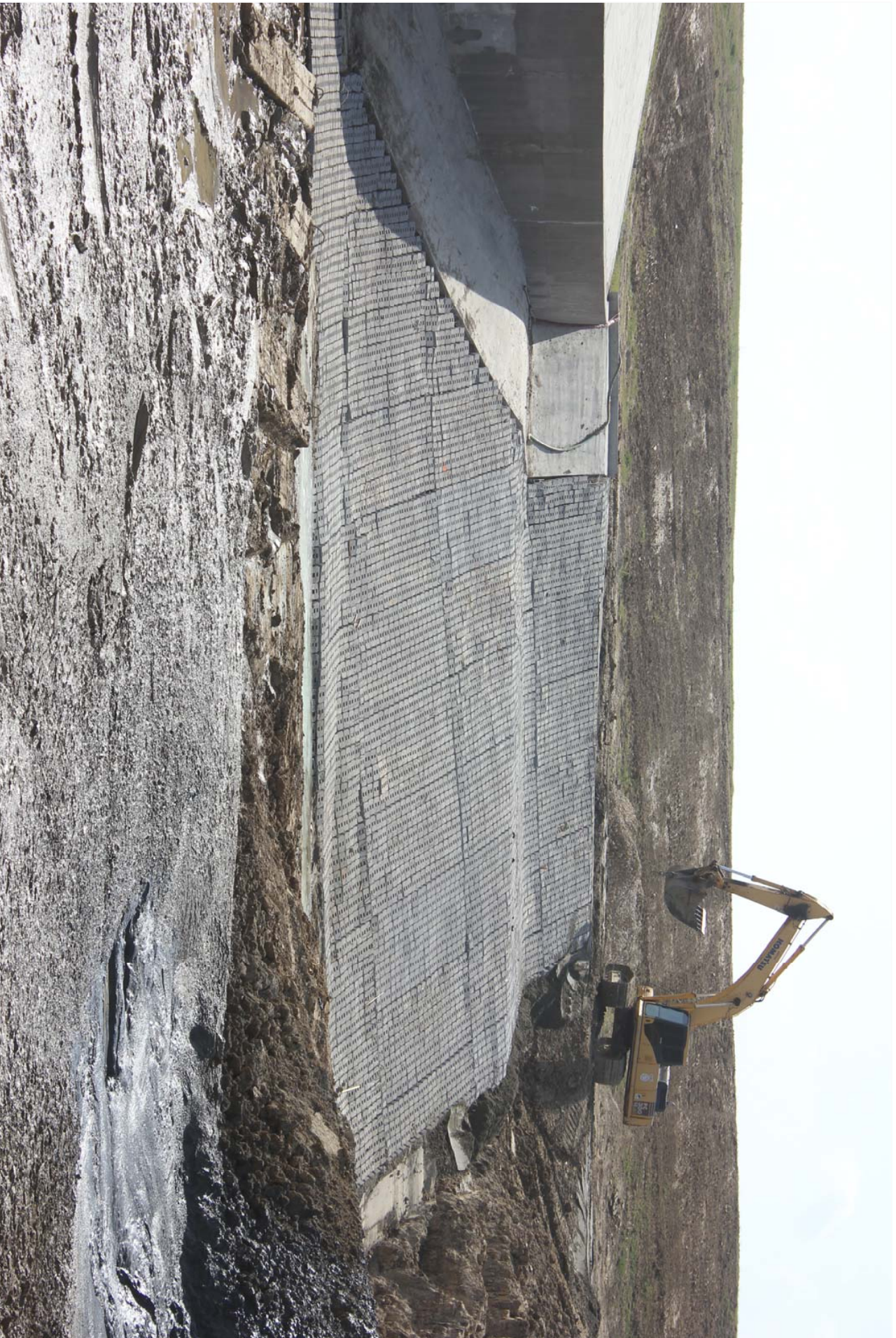
Concrete Mats and Concrete, Southeast Corner of Structure
