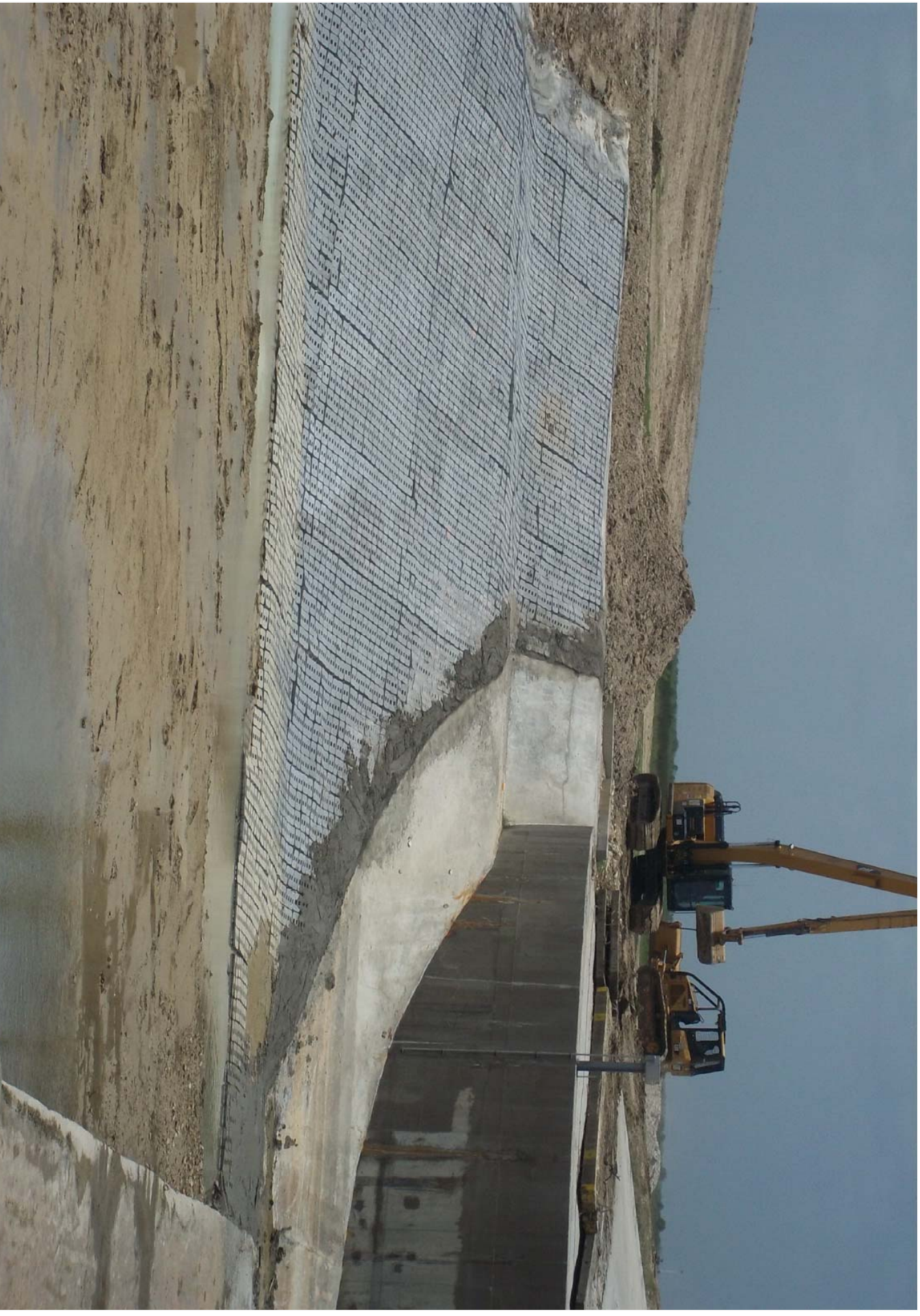
Concrete Mats and Concrete, Southwest Corner of Structure
