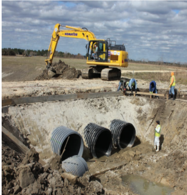
DD6 workers clear and widen a crossing along Byrd Gully.
